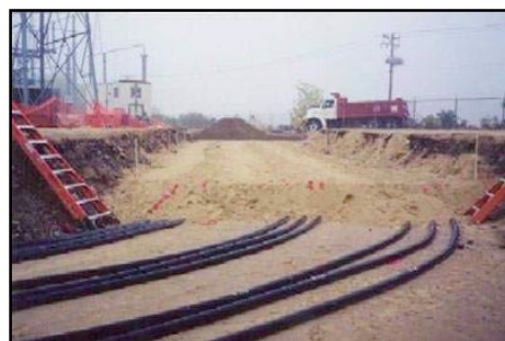
Cable Installation © ENTSO-E/Europacable
