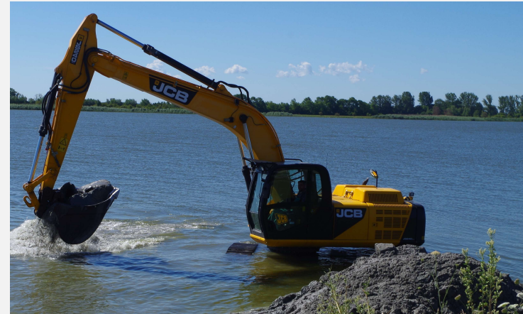
Compensatory measure decommissioning of the Görmitz dam / © 50Hertz
