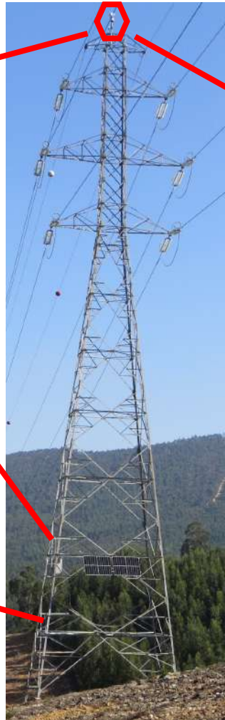
Weather Station For wind speed, air temperature, air moisture, atmospheric pressure, rain fall, bearing, solar radiation and electrical discharges detection (at 2.5m from ground level)
