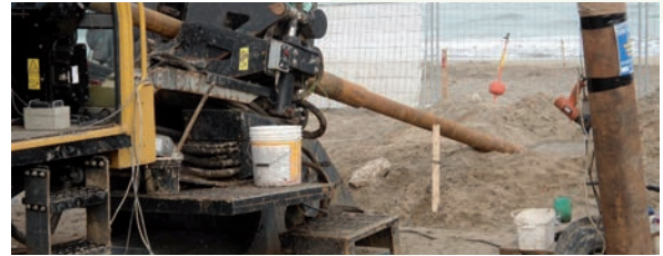
Figure 3: Horizontal directional drilling. Source: Terna
