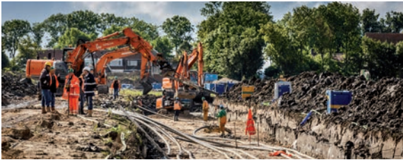
Figure 2: Direct Burial. Source: Europacable
