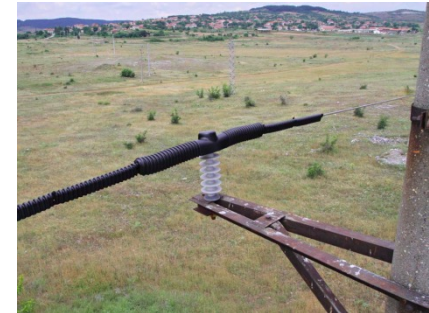
45° angled crossarm + extra perch (upper photo) Insulator cap on 20 kV pole pin-type (photo below)
