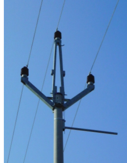
45° angled crossarm + extra perch (upper photo) Insulator cap on 20 kV pole pin-type (photo below)
