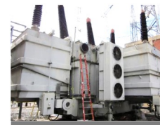
Internal inspection and diagnostic
