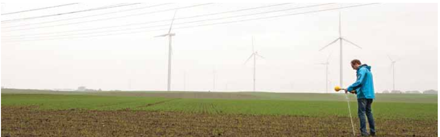
MEF measurements beneath existing 220kV line
