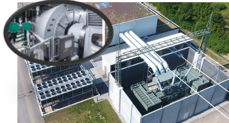
Rotating phase shifter
