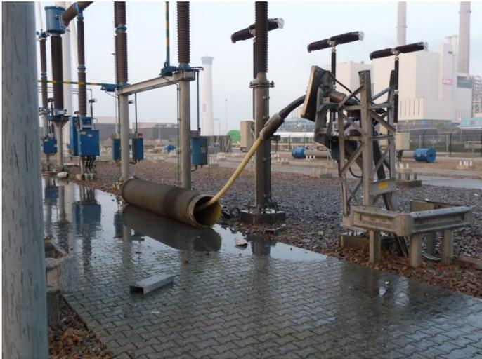
Maasvlakte substation (some 5 years ago): exploded cable termination, incl. oil spillage
