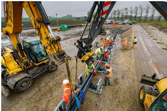
Randstad Northring (2017): cables damaged during drilling under North Sea Canal, still not in service, repair expected in 2020
