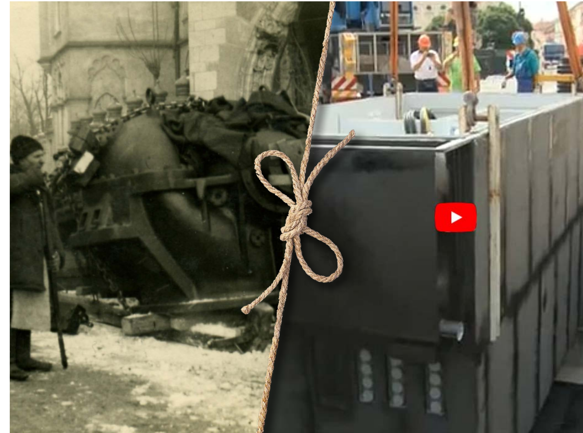
In early last century, the attention of bystanders was attracted by the transport of a steam boiler near the Jakobov palác; early this century, it was attracted by the construction of a unique underground transformer station on Hlavná street. (see also the video about this investment project which was completed under the management of our parent company, VSE Holding).
