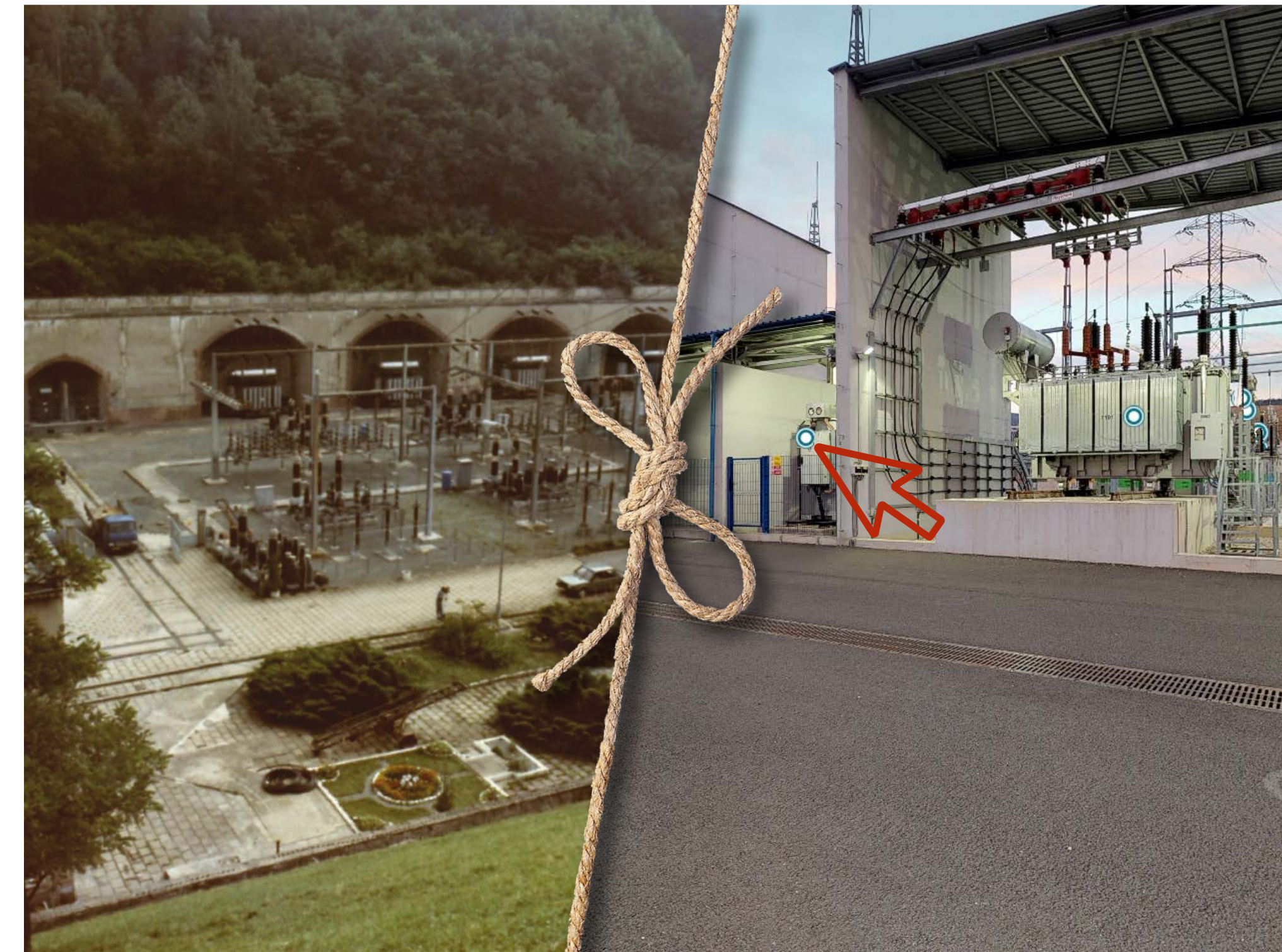
Electric substations have passed significant changes. You can visit one (located in Dobšiná) by means of a virtual visit.
