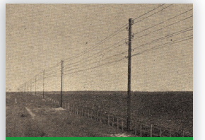
The first power line in the world from Rome to Tivoli, Italy (1882).
