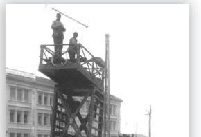
A work team performing operations on pylons
