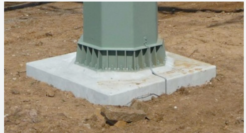
Flat foundation with anchor bolts
