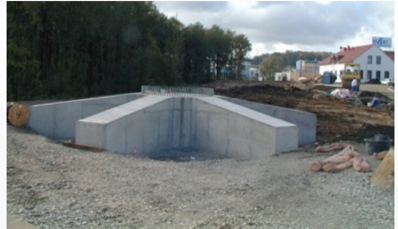
Star shape foundation on rammed pipes
