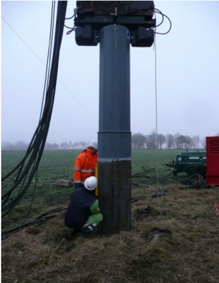
Rammed pipe foundation for suspension poles
