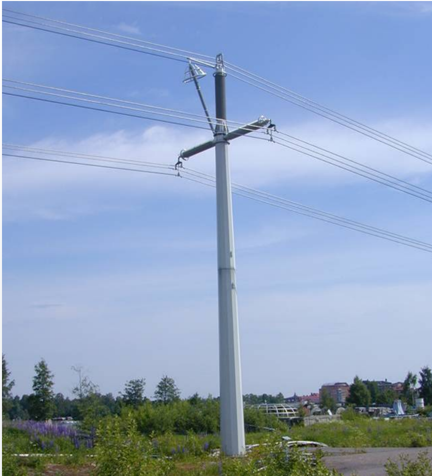
Most Compact Design, Statnett - 420kV with 5m Phase-Distance
